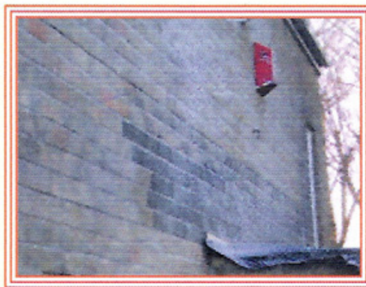
After High Pressure Cleaning
