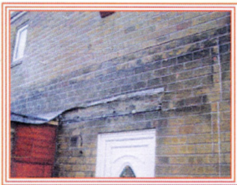
Before High Pressure Cleaning
