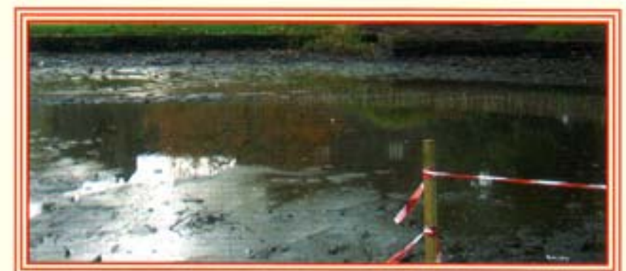
Sludge Lagoon requiring Dewatering
